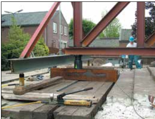
▼ P392 in action with RC256 cylinders.
